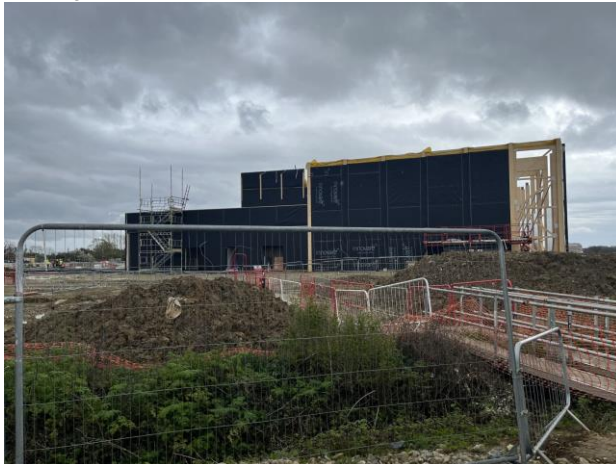
Sports Hall Structure
